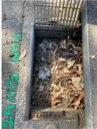
Image 2 – SW Pit 45, unable to visually inspect and measure pipes. Pit has substantial debris. Pit has been joined into the network to quality level C specification.
